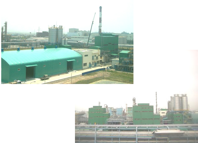
Fig. The foreground of the Fumed Silica Plant
